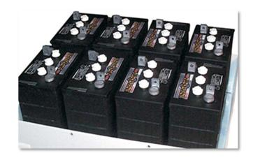
These flooded lead-acid batteries were originally designed for supermarket floor scrubbers.
