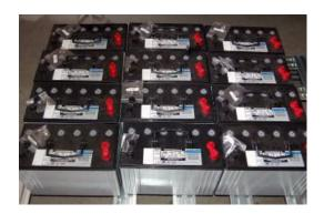
Deep cycle lead-acid batteries have proven to be one of the best (and most affordable) battery types for alternative energy system battery banks for these reasons:
